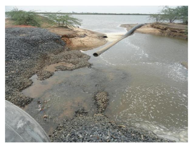
Figure 13: Photograph showing waste water pipeline of thermal power stations discharging effluents into Kandeleru creek.
