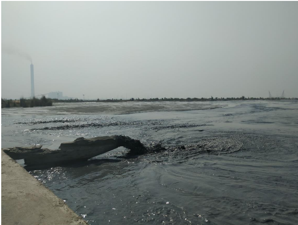
Image 1: Flyash slurry in ash pond of Tenughat TPS, Jharkhand/Photo Credit: Sehr Raheja
