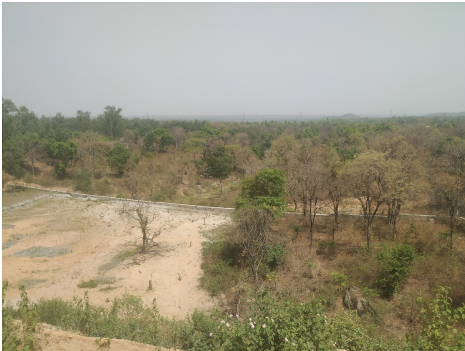
Figure 13: Ash dump near Konar Dam- Boundary wall along the edge of the dump at the bottom; ash reaching the level of the boundary wall and trees in surrounding areas also visible
