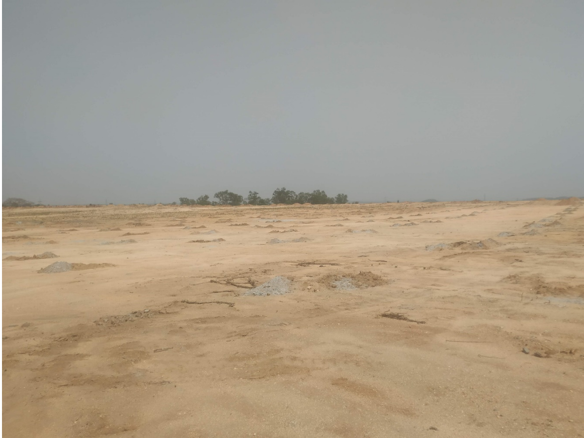
Figure 11: Ash Dump near Konar Dam -Large ash dump covered with soil, with pits at regular intervals for plantation; photo taken from on top of the dump
