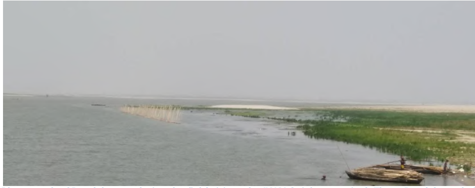
Figure 5: Photograph of Bandals seen during the field visit at the IWAI Gaighat terminal. These Bandals are being used to divert silt away from the navigation channel. Accumulated silt can be seen on the upper right hand side of this picture.
