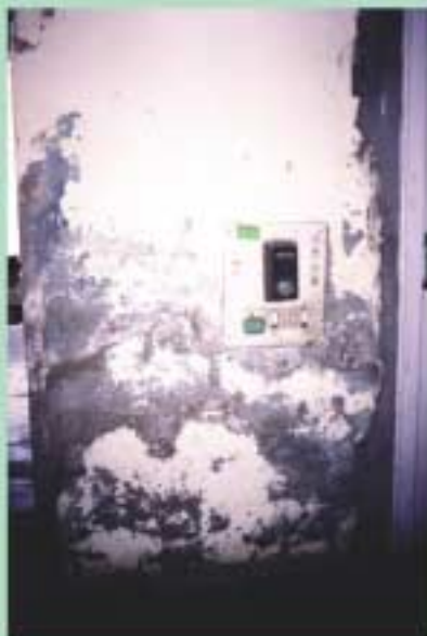
Dampness along the wall at a house in Malout town, District Muktsar, Punjab leading to peeling off of the paint and plaster. Waterlogging has impacted about 70% of the houses in this town, and houses require repair at regular intervals.
